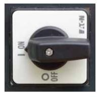
Switch ON the selector. The cabinet starts the cooling cycle.
